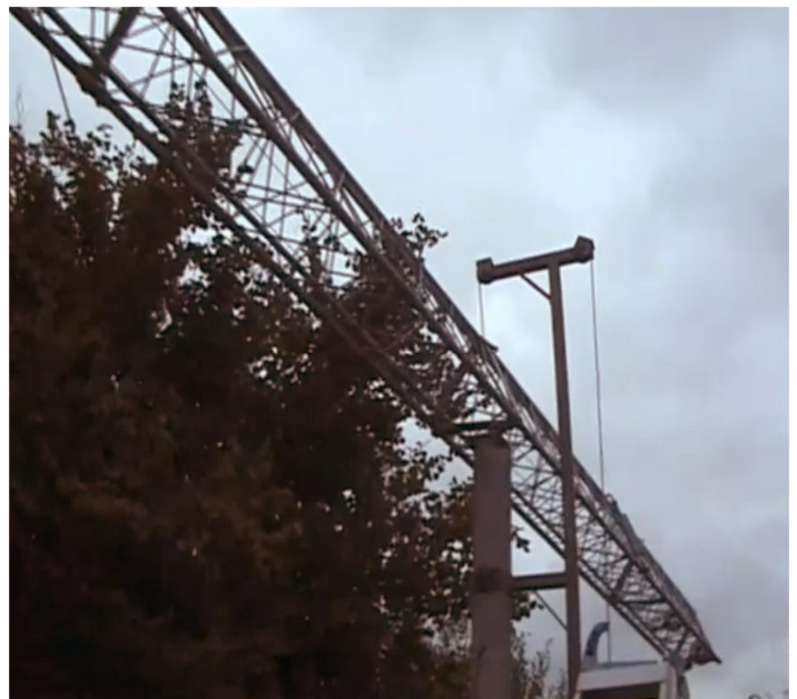
Lifting the tower into position onto the pole
