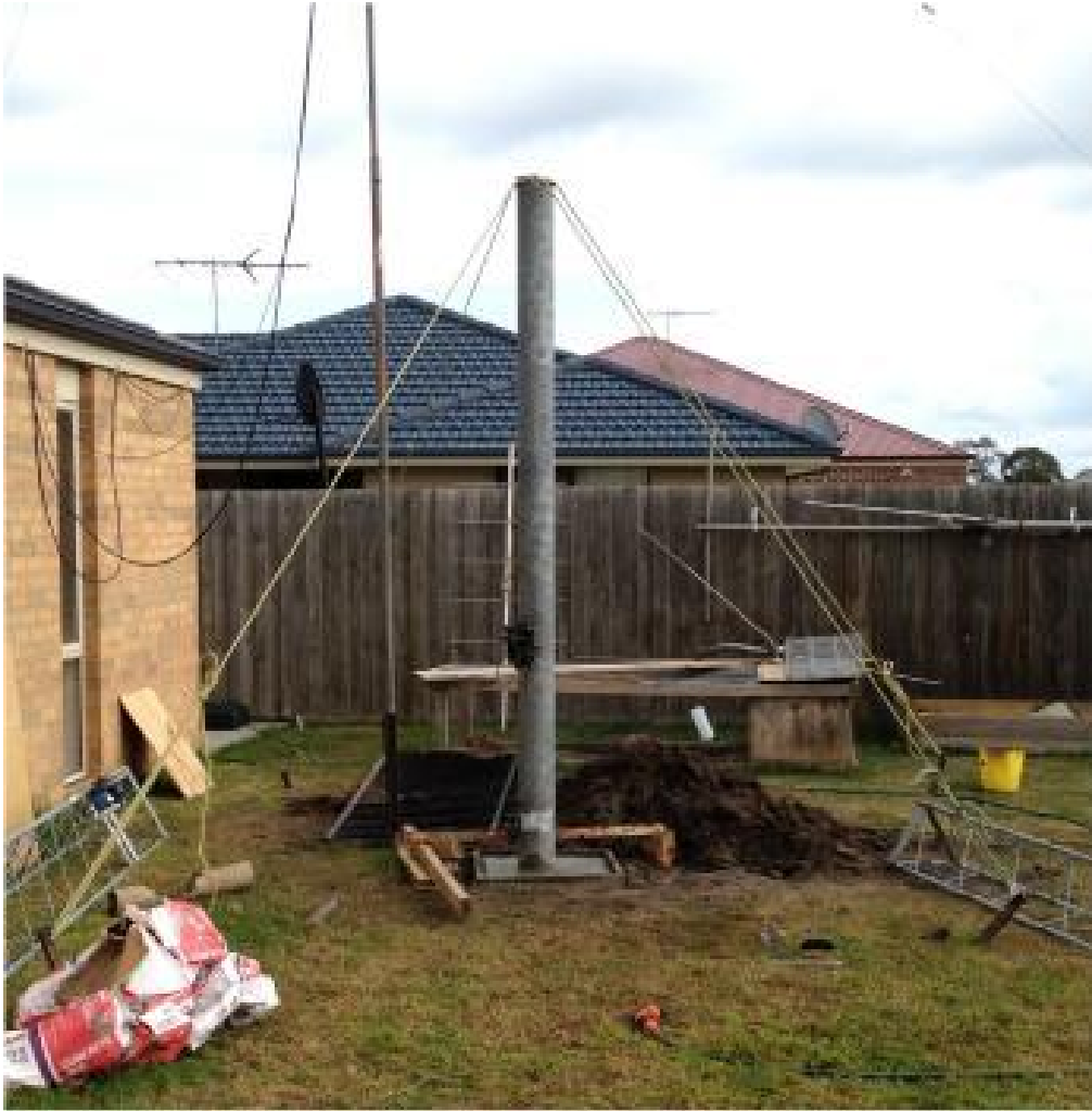
The pegged out pole, waiting for the concrete to set.
