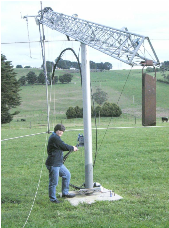
A counterweight makes tilting the tower easy
